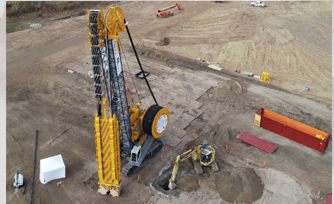
Trench cutter bulk sample rig
